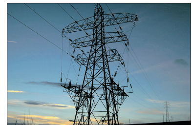
Utilities: maintenance and minor works
